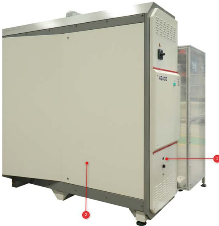
Figure 5-15 Incoming power supply cable inlet
