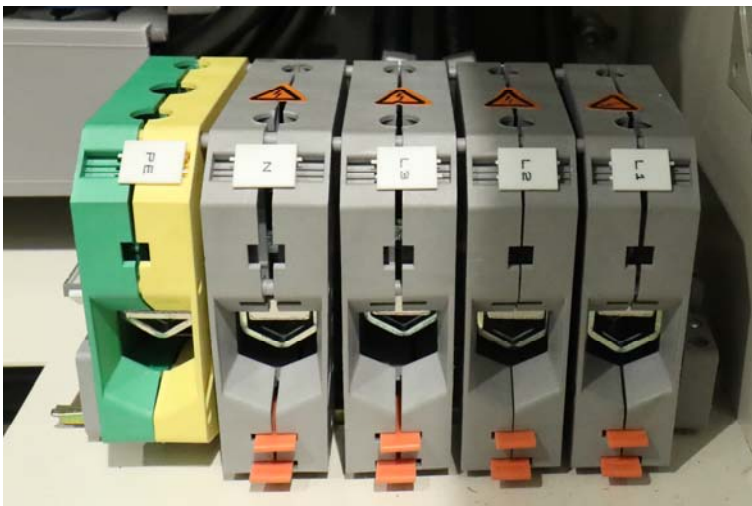
Figure 5-17 Connecting incoming power supply cable
